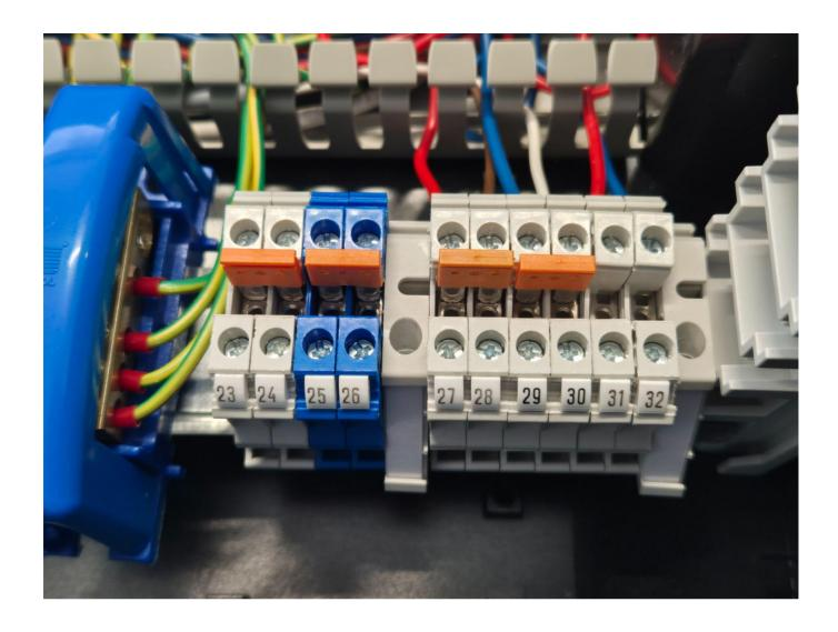
To reattach markings onto terminal connectors squeeze them in place with the help of the flat head screwdriver.
