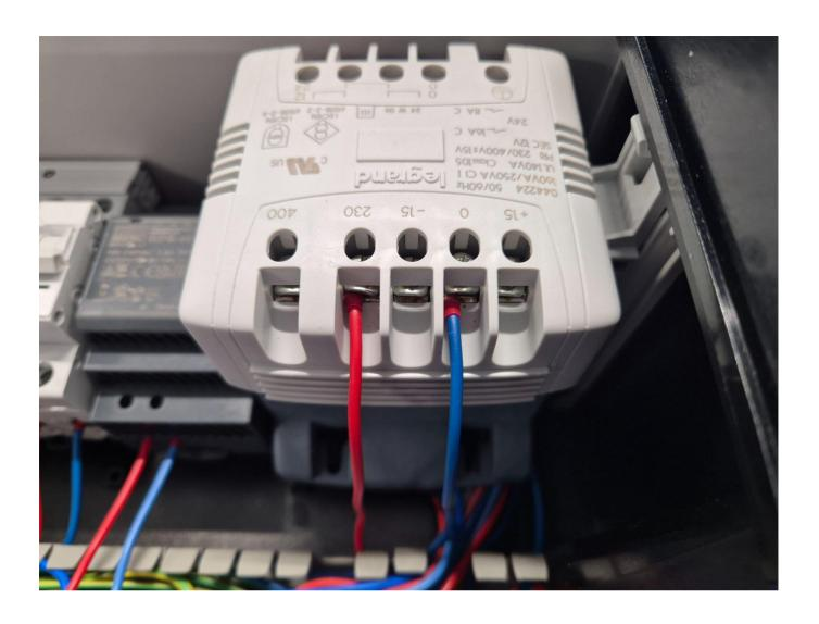
The next step is to loosen screw terminals on transformer 230 VAC marked as 230 and 0 without pulling wires out.
