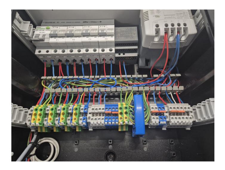
The next step is to route wires in the cable channel and close the lid.
