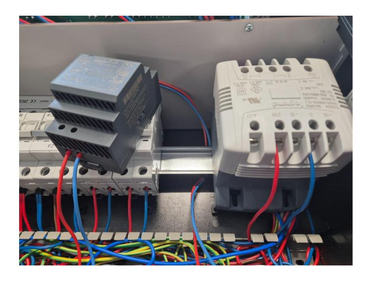
The power supply should be placed between miniature circuit breakers and transformer 230VAC/12VAC
