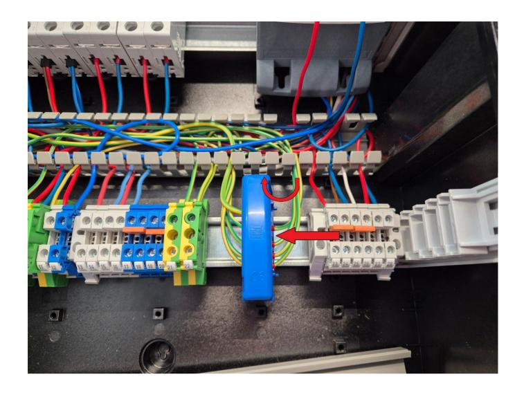
Next step is to slide protective earth terminal to the left and take right side wires out of the cable channel ribs and move them to the left.
