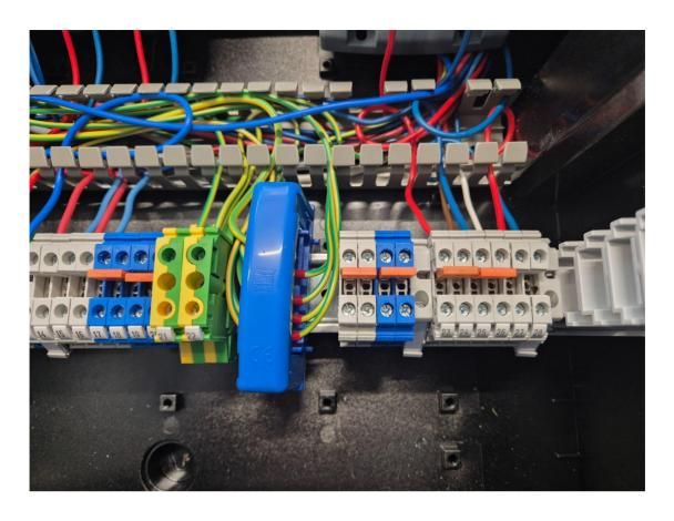
The next step is to install terminal connectors (grey x 2 and blue x2) as shown on the photo above.
