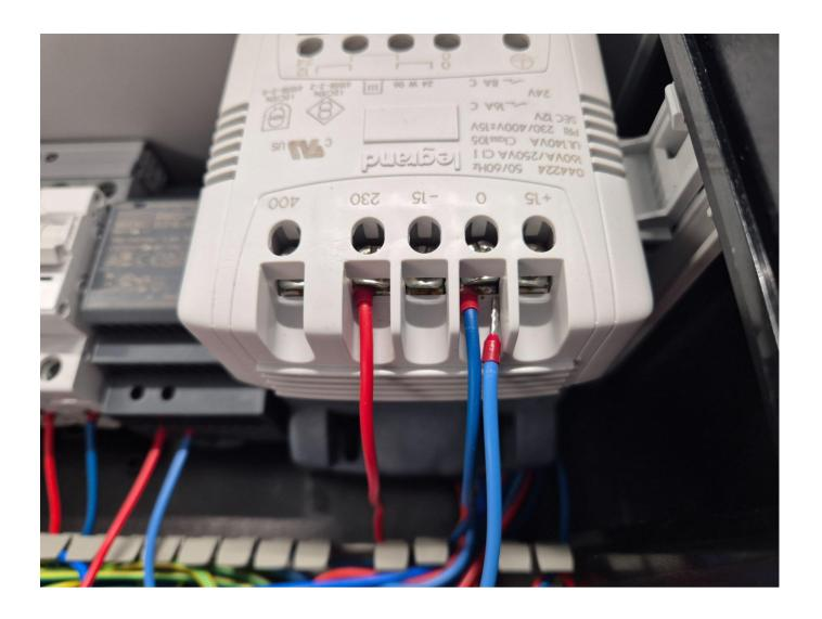
Connect wires coming out of the bottom of the power supply 230VAC to the transformer. Red wire to screw terminal marked as 230 and blue wire to terminal marked as 0. Secure connection by screwing in phillips head screw.
