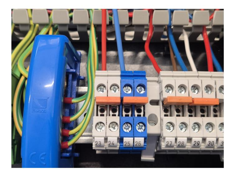
Route top wires from the power supply under transformer into the cable channel and connect them to terminal connectors.
