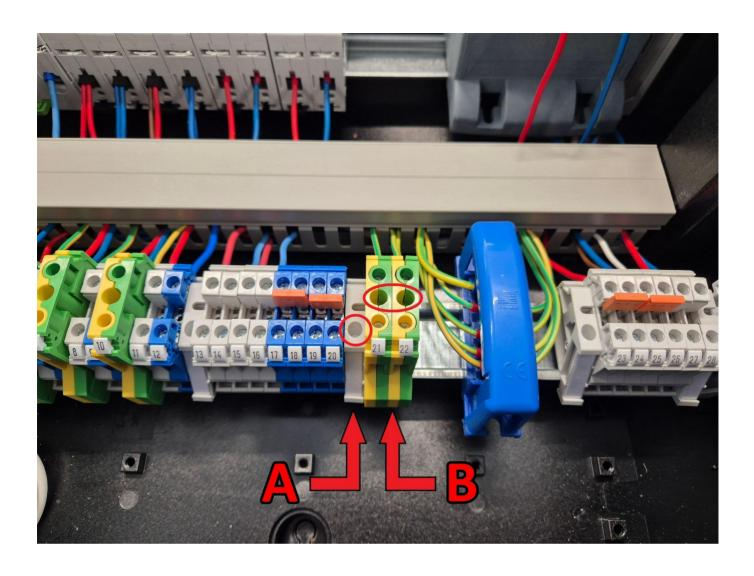
First, loosen terminal connector middle screws number 21 and 22 (marked on photo as B).
